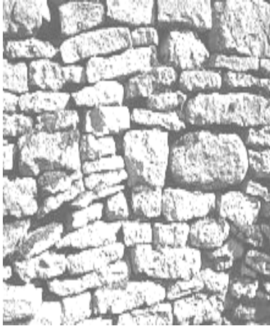
Dry-stone retaining wall:
