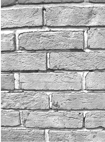
A brick building wall:
